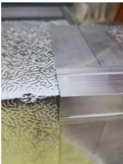
After the ventilation channels are connected, the cover cap can be placed around the corner to ensure a beautiful invisible finish of the connection. The corner cover cap can be fastened with sealant/glue onto the corners or with some self-drilling screws.
